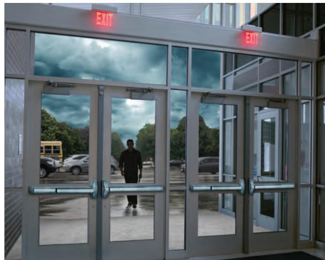
verts to secure mode when electricity is removed, which prevents entry at every door equipped with this type of device.
